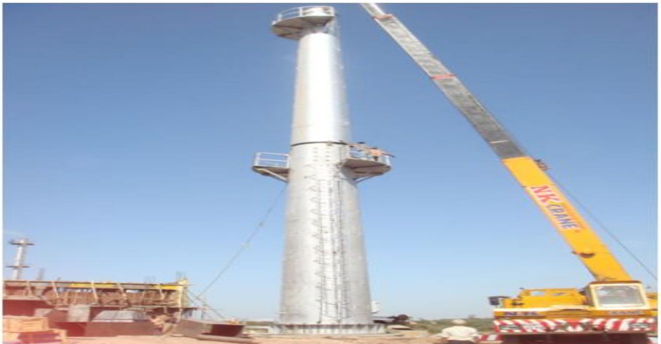
CHIMNEY ERECTION
