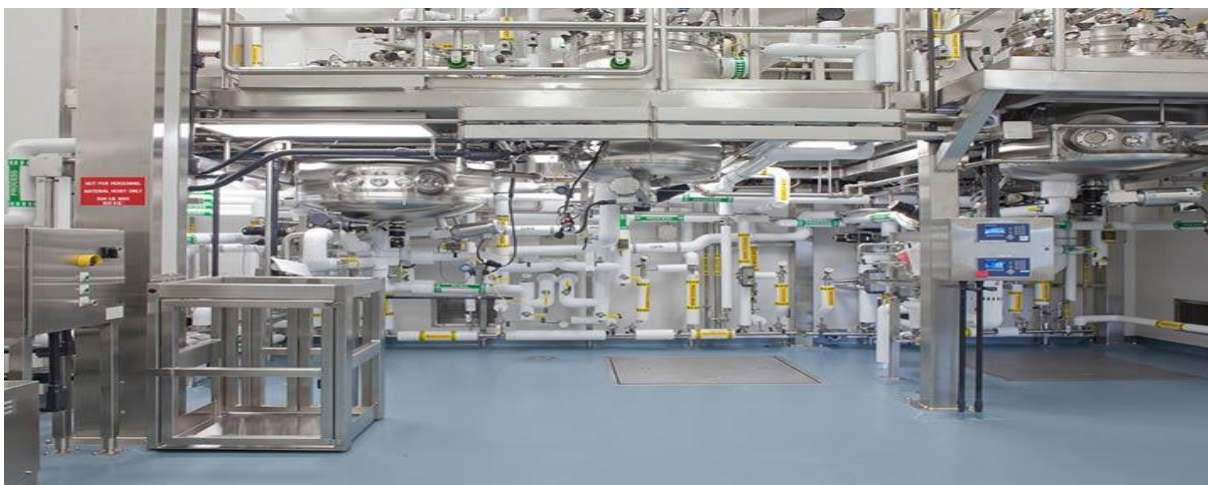
SS PIPING WITH INSULATION
